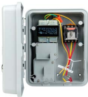
Pump Start Relay
