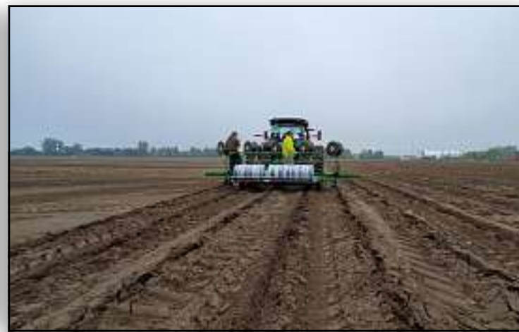
The main line is installed below the frost line.
