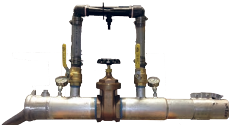
Assembled 1 1/2" Mazzei Injector on 4" Wade Rain Manifold
